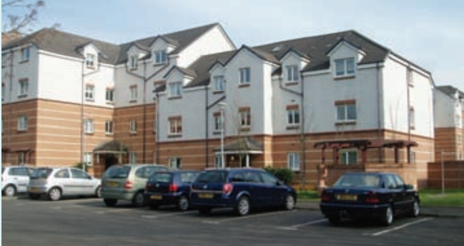
Our new build at Dairsie Court.
