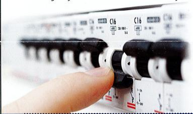
the switches have changed position i.e down instead of up generally the Residual Current Device (RCD) will have tripped and cannot be reset.
