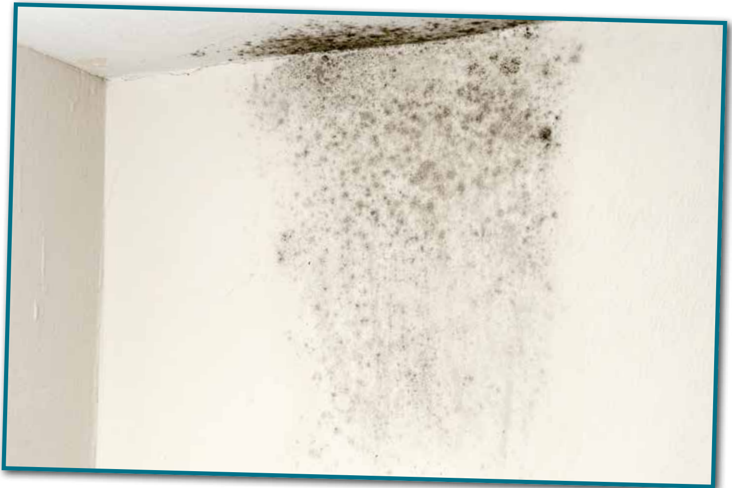
Example of mould growth if untreated
